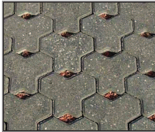
PLATE 6.3 – TYPICAL PERMEABLE PAVERS
