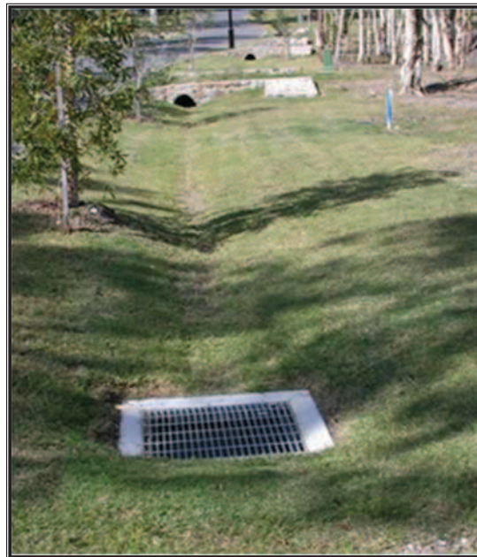
PLATE 6.1– TYPICAL GRASSED SWALE
