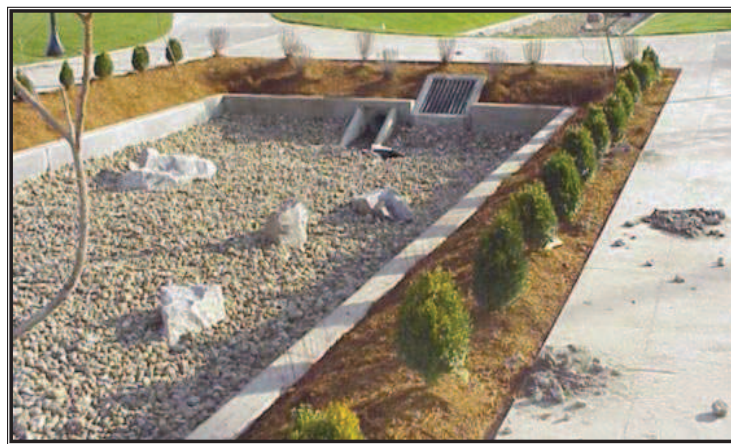
PLATE 6.2 – TYPICAL SAND FILTER
